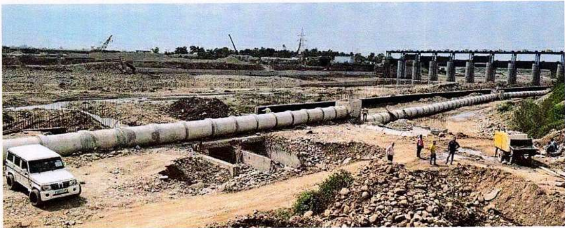
Picture showing Interceptor Drain On Right Bank
