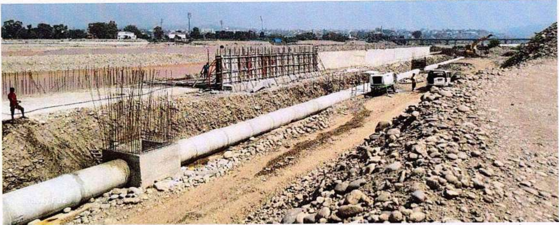
Picture showing Interceptor Drain On Left Bank
