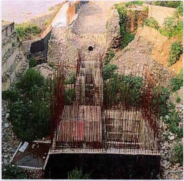
Under Construction Intermediate Pumping Station, Tawi Riverfront-Left Bank (executing agency JSCL)
