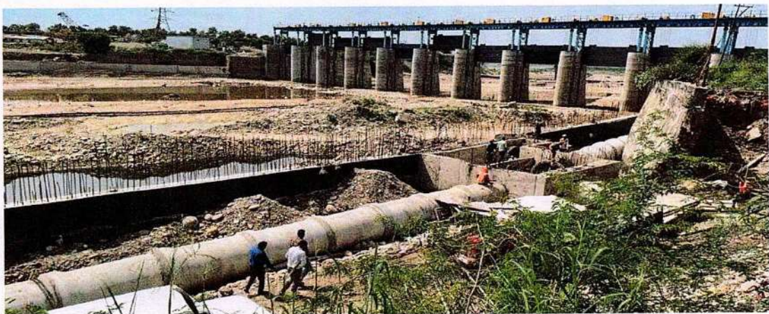
Picture showing Interceptor Drain On Right Bank
